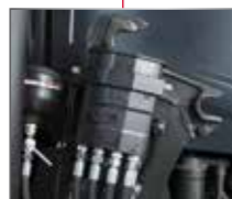
On the MX loader control valve
